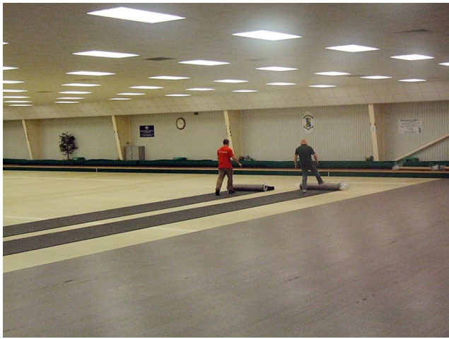
This was taken in 2007 when the present underlay was being laid
